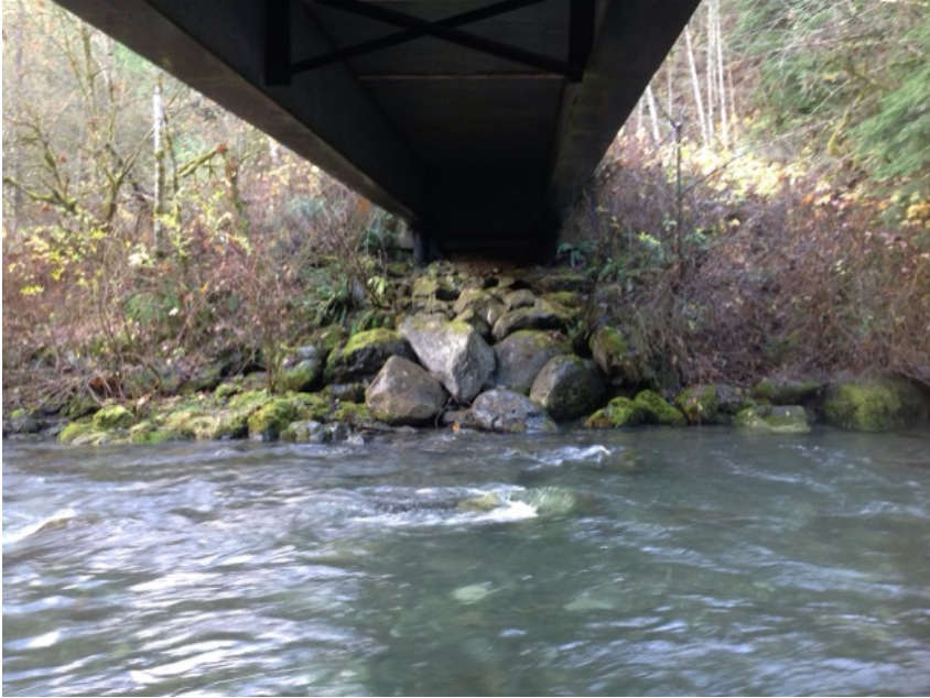
Right Bank Abutment when facing downstream
