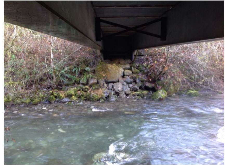
Left Bank Abutment when facing downstream
