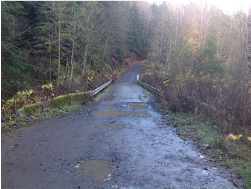
Approach from Right Bank when facing downstream
